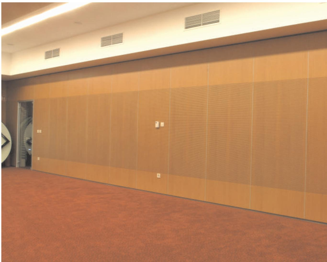
*OdAcoustic line of products consists of panels realized with deadening materials that allows high acoustic performances. They are easy to assemble, easy to maintain and allow the re-use of materials. Different kind of drillings and millings are available in order to obtain the best sound proofing results in all the range of frequencies.*
